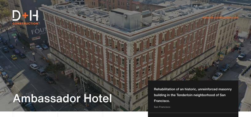
The building will undergo a seismic upgrade comprised of a steel horizontal bracing system, new concrete foundations and concrete reinforcing walls, and exposed steel frames adjacent to the rear courtyard brick façade. Existing street facing storefront steel brace frames will be structurally enhanced to strengthen the existing structural deficiencies.
