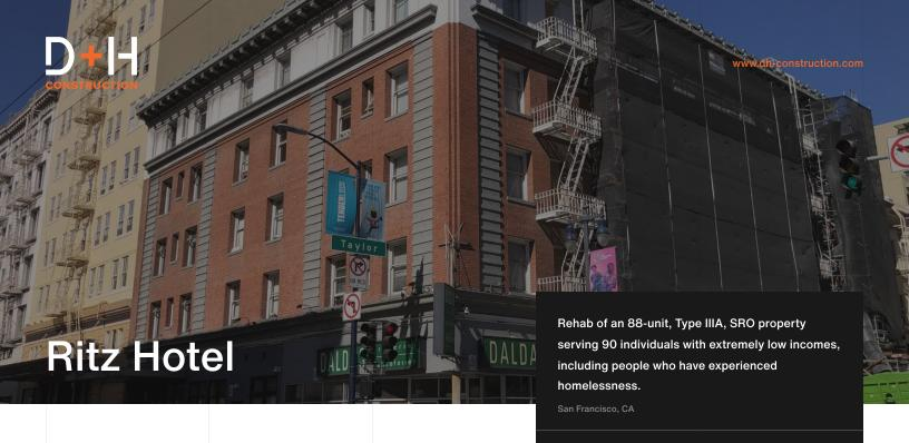
Work includes seismic upgrades, unit ADA improvements, installation of a sprinkler and ERRCS system, unit and common area bathroom upgrades, electrical upgrades, energy improvements and the addition of a community room.
