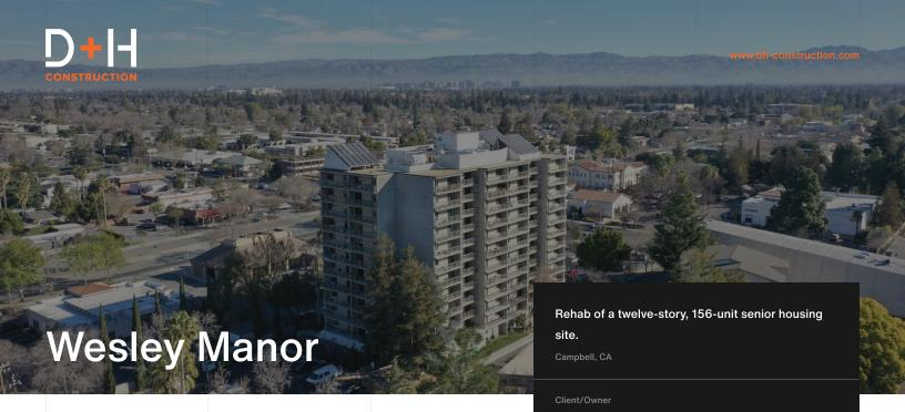
Work is driven by seismic upgrades, which use both shotecrete and Fiber Reinforced Polymer (FRP). There will be new finishes, MEP upgrades and modifications in both unit and common area interiors. Exterior and site work is limited to areas directly affected by the seismic improvements.
